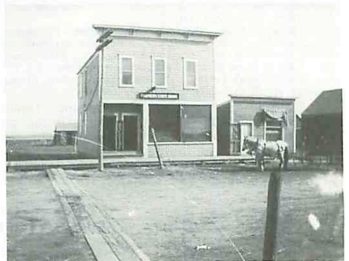
Note board crosswalks
