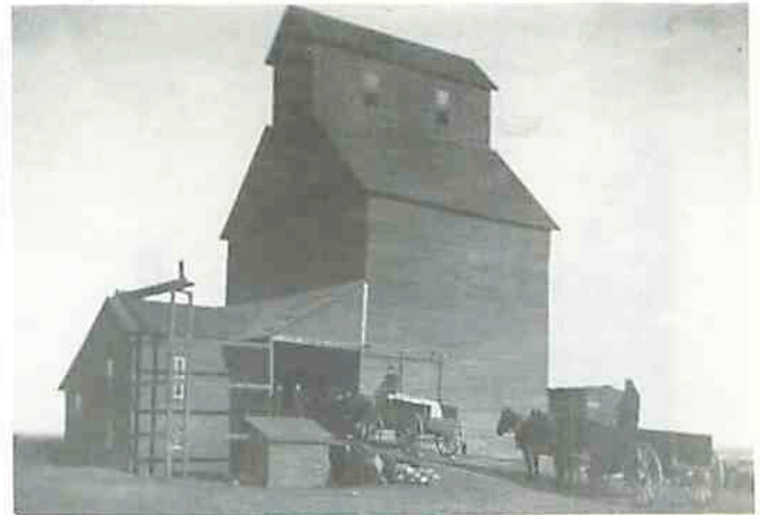
Chase Elevator - First elevator in Almont
